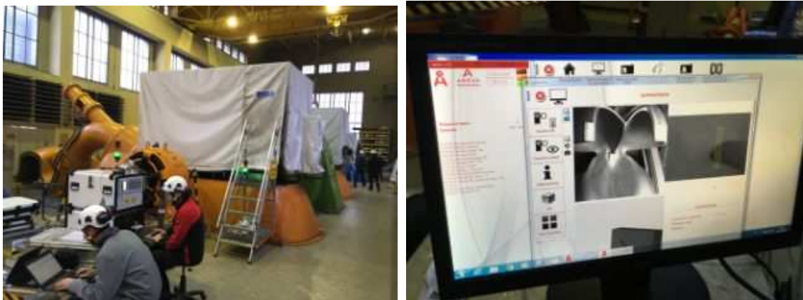
Fig. 11: the PTC system under laser protection tarp during Pelton onsite inspection - Periodical check of the system before inspection with ATHENA software interface
